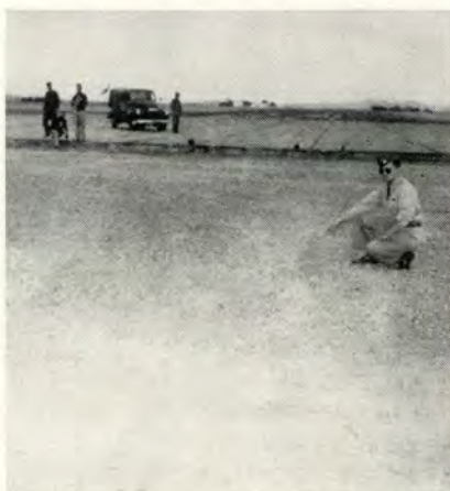
Throttle applied too late. Landed 50 feet short in construction area. Left, note impact marks. Plane rolled to edge of runway and both main gears sheared. Right, see lip.
