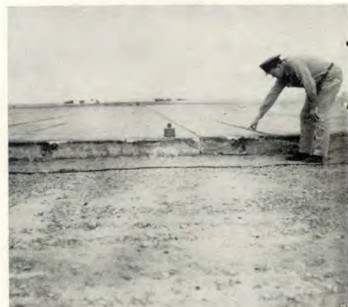
Throttle applied too late. Landed 50 feet short in construction area. Left, note impact marks. Plane rolled to edge of runway and both main gears sheared. Right, see lip.
